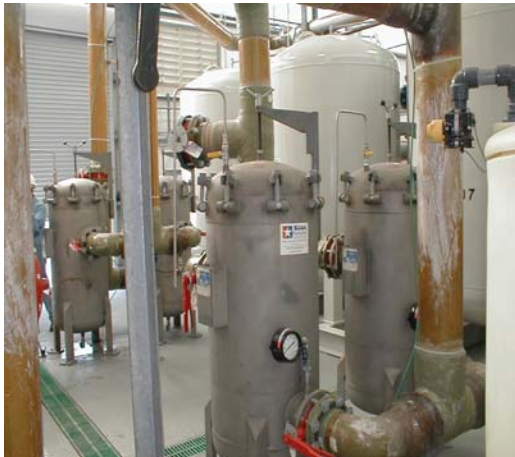
Figure 2: SS Filters were provided with a design capacity of 500 gpm each.
